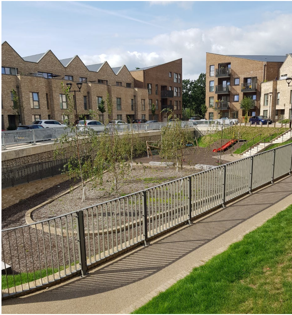
Image: Completed Blocks G2, G3 and H4
